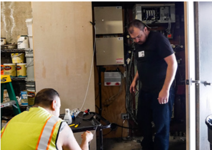
Monkeybrains Lead Engineer Mason Carroll (R) watches as DT technician Alex Hernandez prepares to fuse fiber.
