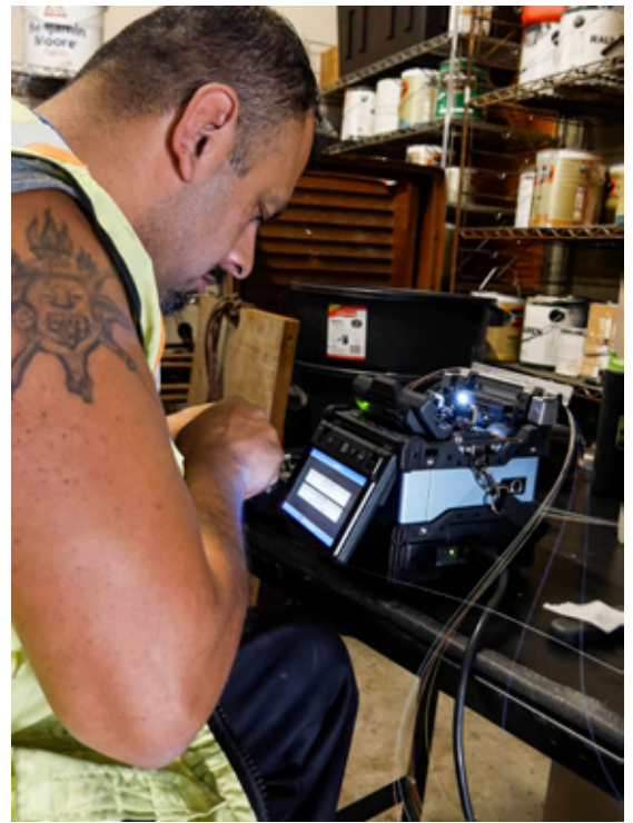
SF Department of Technology technician Alex Hernandez fuses fiber at St. Mary's shelter.
